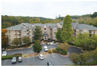
Example of an apartment complex that may be found along a Suburban Corridor. ▼
