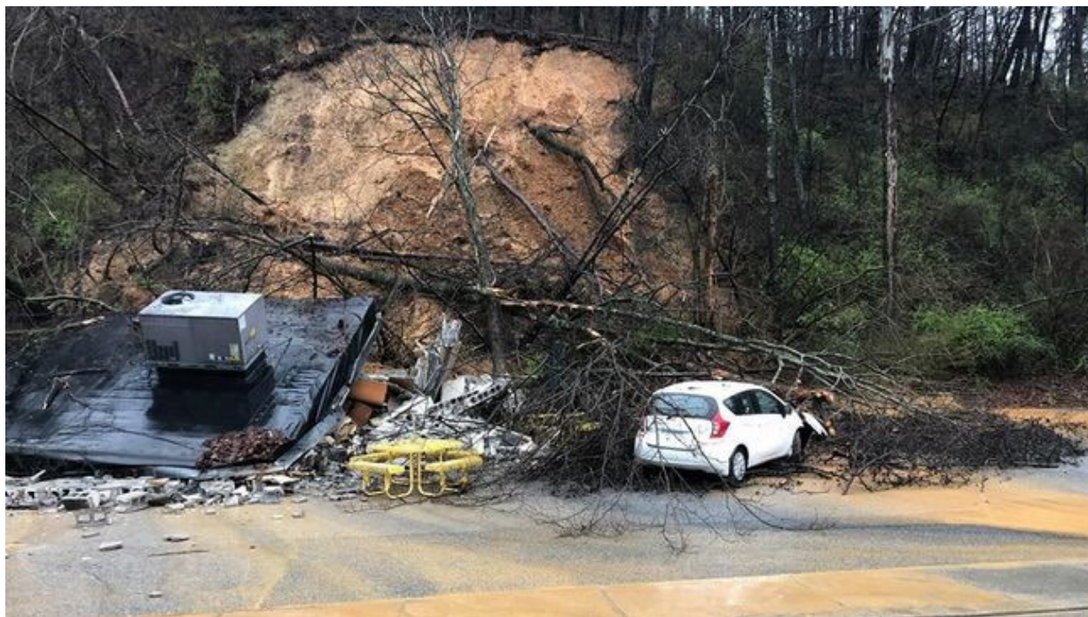
Mudslide that destroyed the former Subway restaurant on Signal Mountain Road in 2019.
